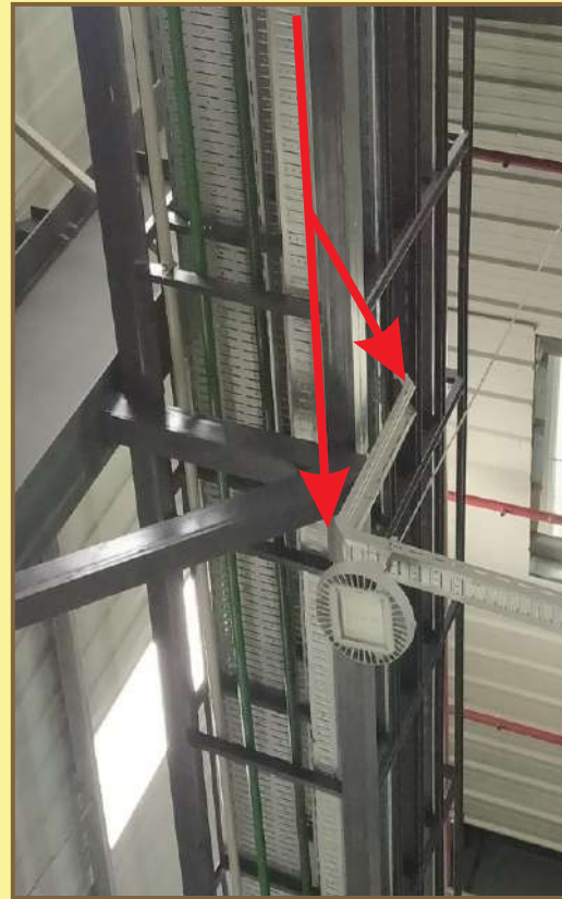
Cable Tray Bends & Elbows as per requirement
