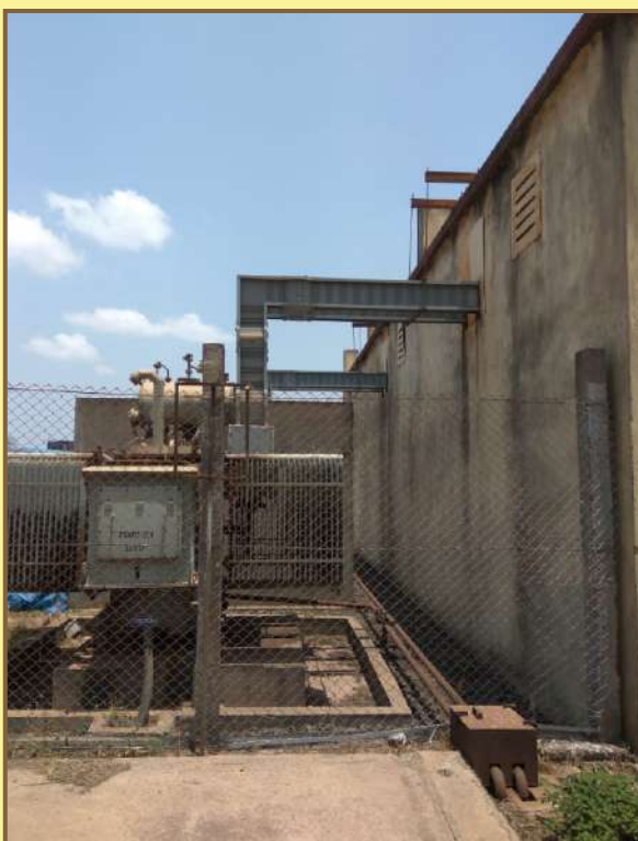
Installation & Commissioning of 2500 x 2 Sandwich type Bus Duct
