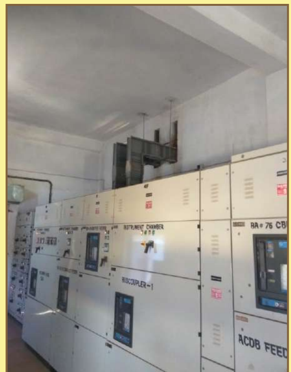
Termination of Bus Duct to LT Panel
