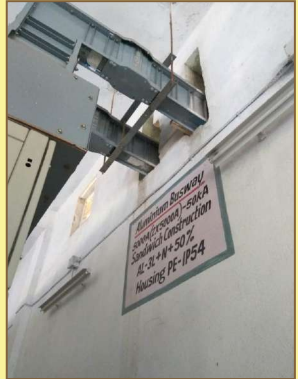
Installation & Commissioning of 2500 x 2 Sandwich type Bus Duct
