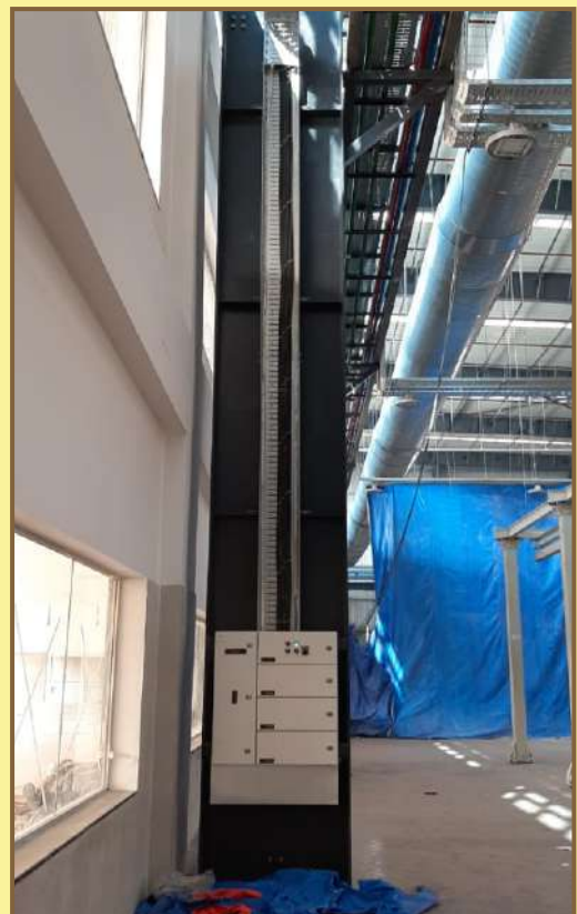
Installation & Commissioning of Sub Distribution Panel
