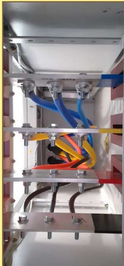
Termination of LT Cables
